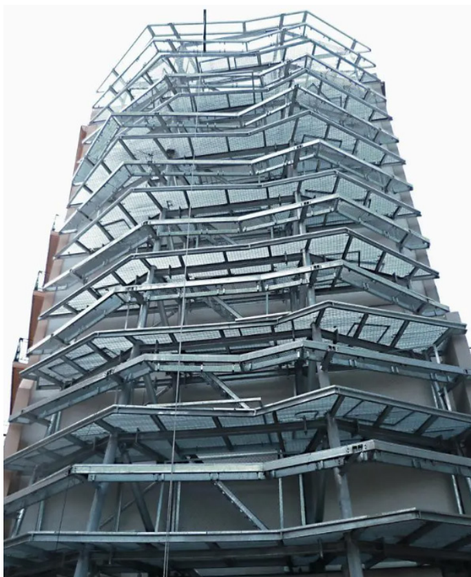
Figure 55: Prefabricated galvanized steel structure Source: Capella Garcia Arquitectura
